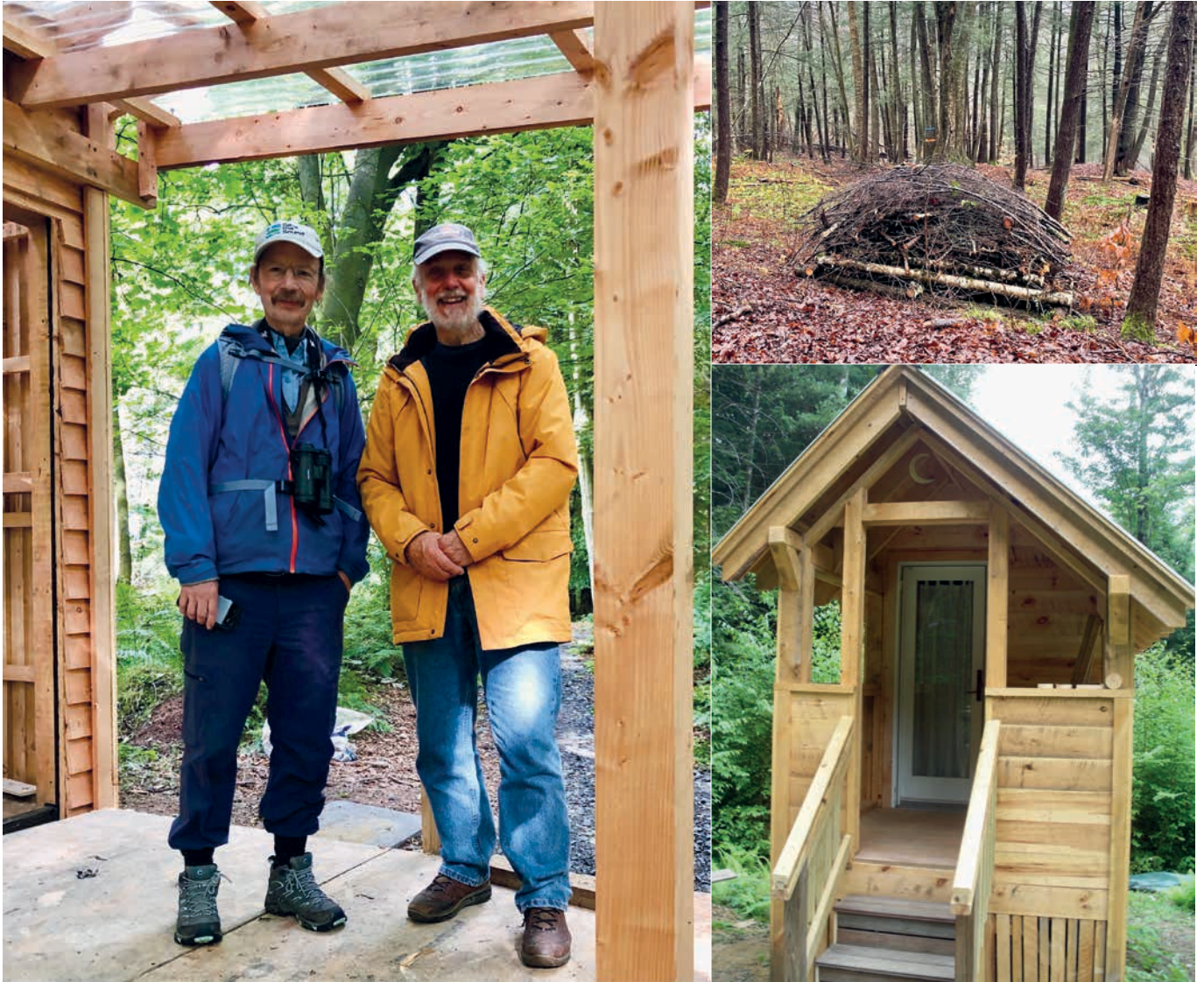
John (left) with Andrew at Hut of Wellbeing during construction; brush pile on John's land for habitat; the pooh palace! Photos: John Sargent.
