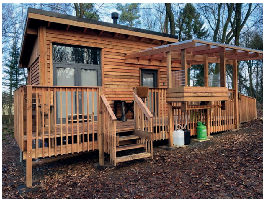
Hut of Wellbeing in its finished form. Photo: Andrew Johnson.
