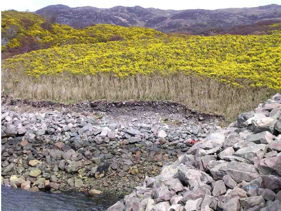
Figure 3. Dense and extensive monotypic Gorse growing on foundation infill of the Skye Bridge, Lochalsh (2006). Five years later this stand is now much more open with an understorey of little trees, herbs and bryophytes, and several saplings are already overtopping the Gorse.
